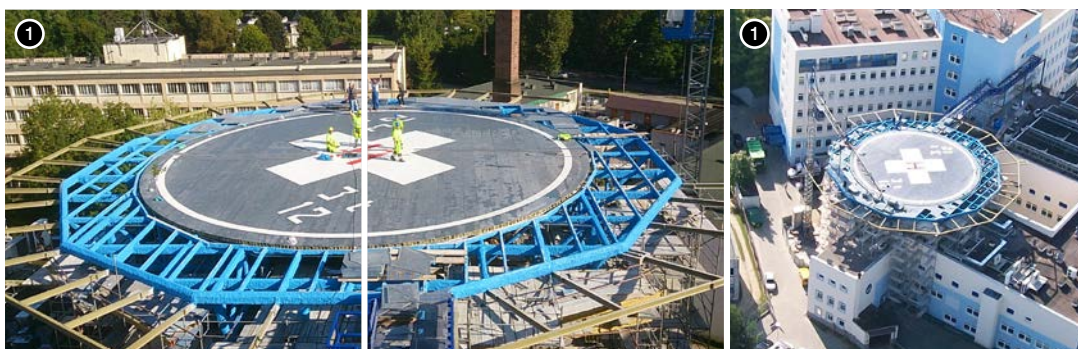
1. Helipad on the roof of the Home Office Hospital - Olsztyn, Poland.
