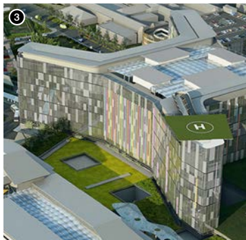
3. Modern hospital complex – Glasgow, Scotland. System KAN-therm Inox
